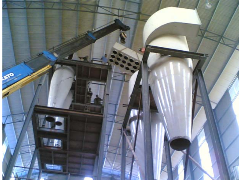
Photo 17: Silos are being installed at the FELDA Bkt Sagu OPF Plant.
