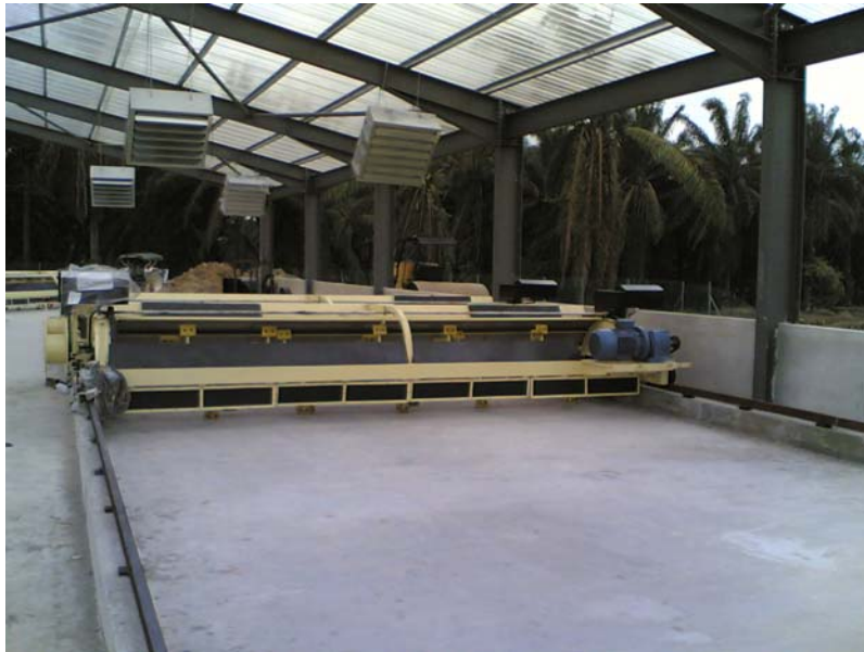
Photo 15: The OKADA System is being installed and tested out.
