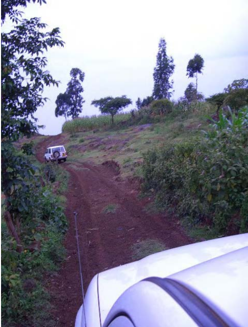
Feeder road to Koibei Location, Endeless Division, Trans-nzoia District
