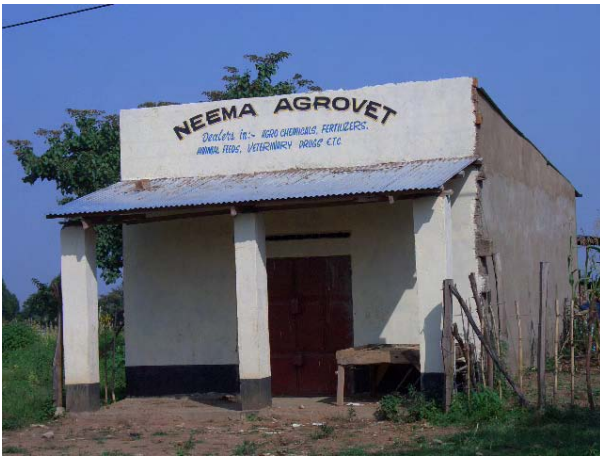
Outlet of agrochemicals, Namubila location, Malakisi division
