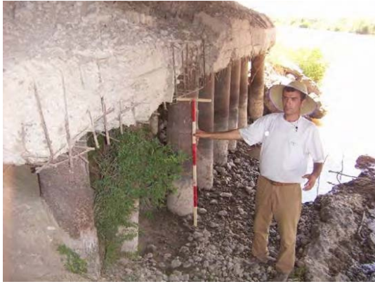
Fig. 2-9 State of the Abutments of Existing Bridge No. 7
