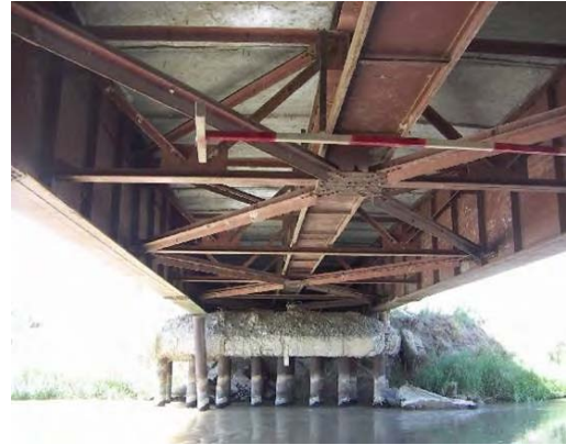
Fig. 2-10 State of the Abutments of Existing Bridge No. 7
