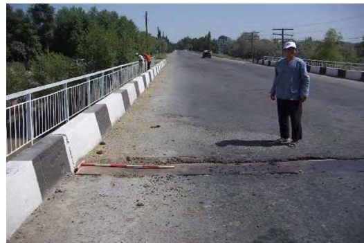
Fig. 2-7 State of Expansion Joints at Existing Bridge No. 7
