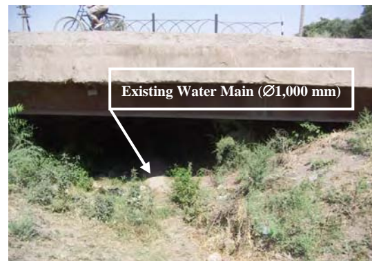
Fig. 2-11 Existing Water Main (Ø1,000 mm) under Existing Bridge No. 13
