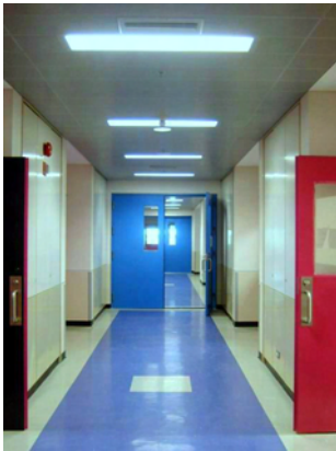
Doors indicate the temperature management
