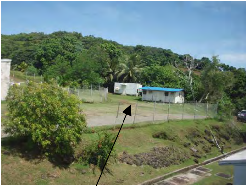
Potential site for new power house
