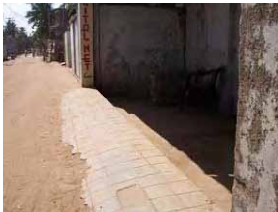
Photo 6.4.2 Prevention of Storm Water Intrusion by Embankment at the Entrance of a House
