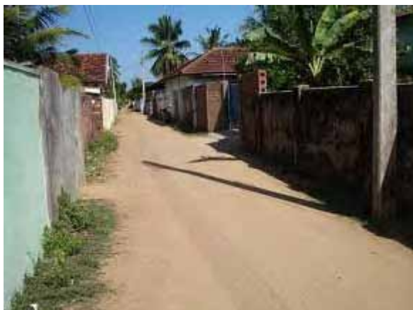
Photo 6.4.1 Unpaved Road without Drainage Facilities in Project Area
