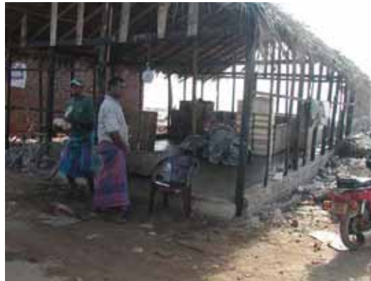
Photo 6.5.11 Fish Handling Shed Restored after the tsunami
