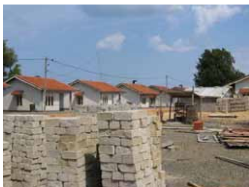
Photo 4.3.5. Site of Cement Block Making
