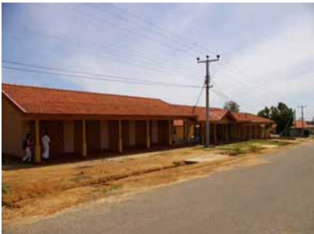
Construction of Hijra Nagar JSFV (Shopping Complex, October 2007)
