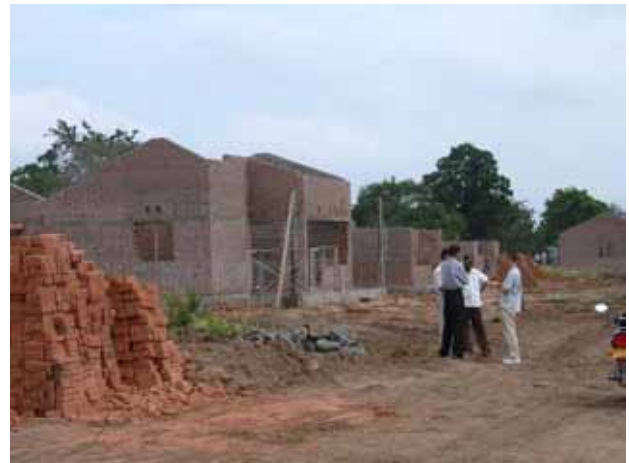
Construction of Hijra Nagar JSFV (February 2006)
