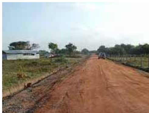
Photo 4.3.11 Access Road, Veloor FCS, Trincomalee
