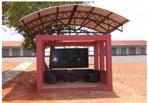
Construction of Konesapury JSFV (Bus Stop and Shop Building, October 2007)
