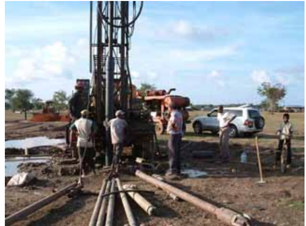
Construction of Iqbal Nagar JSFV (February 2006)
