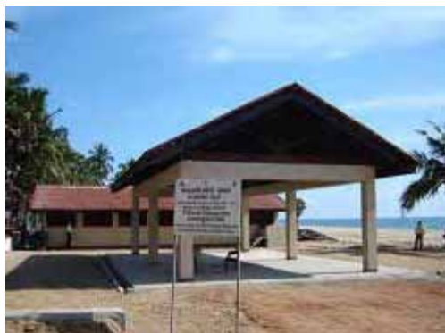
Photo 4.3.10 Lockers and Fish Handling Shed, Hidayafuram FCS, Ampara
