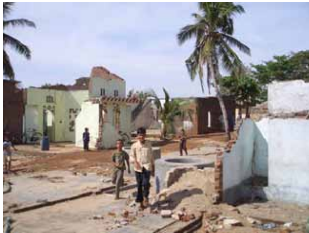
Damaged houses in Sainthamaruthu, Ampara (October 2005)
