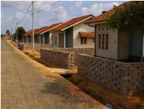
Construction of Iqbal Nagar JSFV (October 2007)
