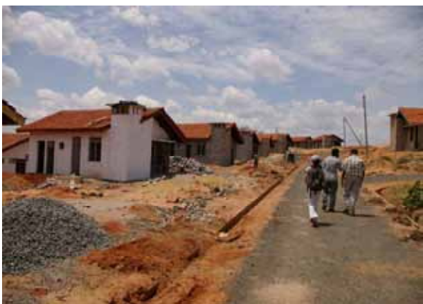
Construction of Konesapury Site (Red Cross House, October 2007)
