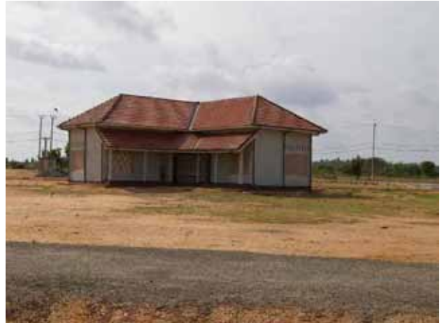
Construction of Iqbal Nagar JSFV (Pre-School, October 2007)
