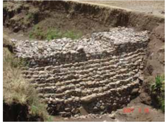
Soil and Silt Dam
