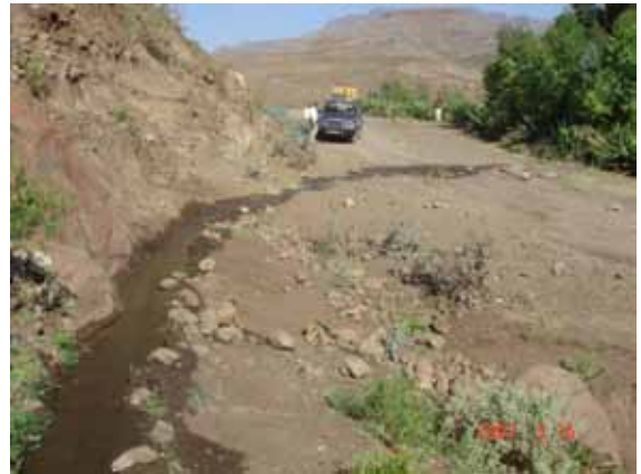
Water Diversion (下流側)
