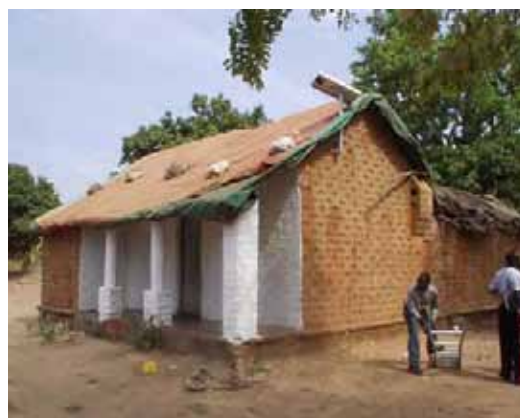
Figure 9-5 A house equipped with a Solar Home System in Lundazi
