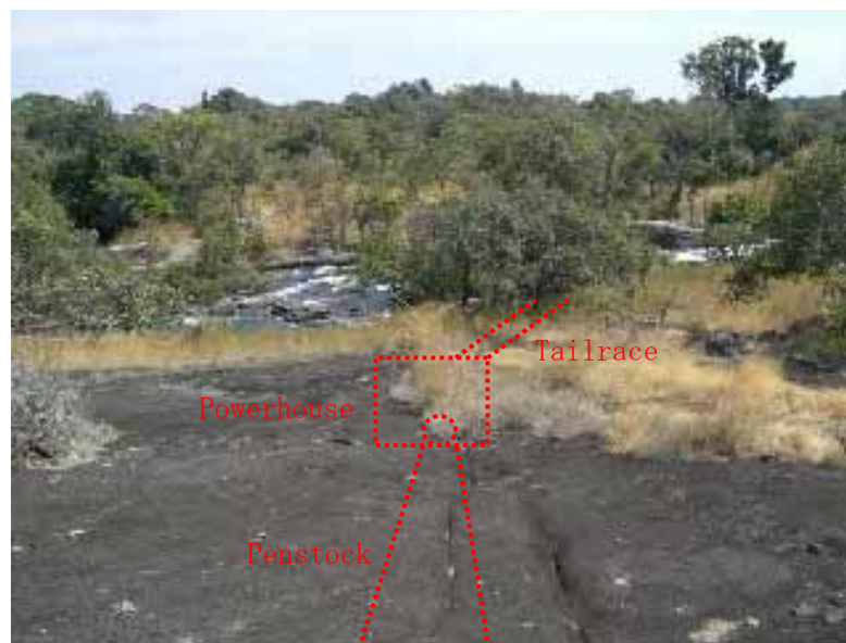
c) View from head tank to powerhouse
