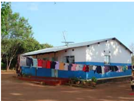
Figure 9-3 A House Equipped with a Solar Home System in Chipata
