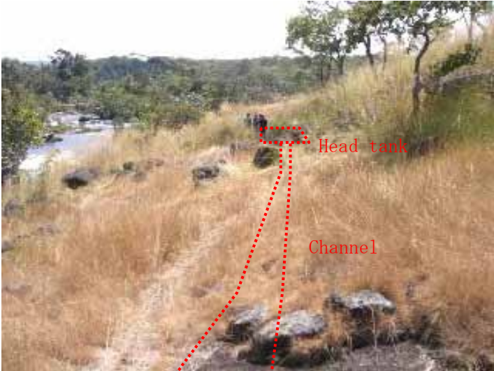
b) Water channel on the right bank
