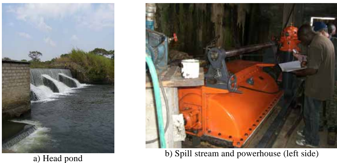
Figure 3-12 Pictures of Mangongo Hydropower Plant
