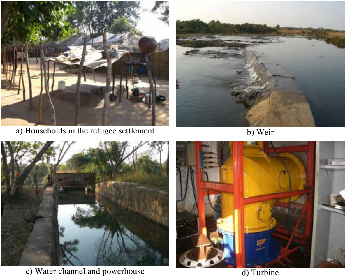
Figure 3-11 Pictures of Luena River Hydropower Plant
