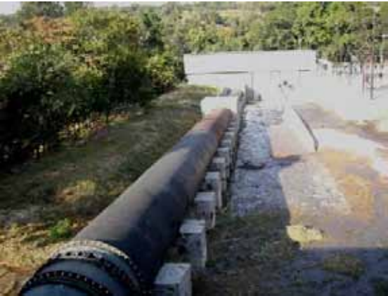
c) Penstock and powerhouse
