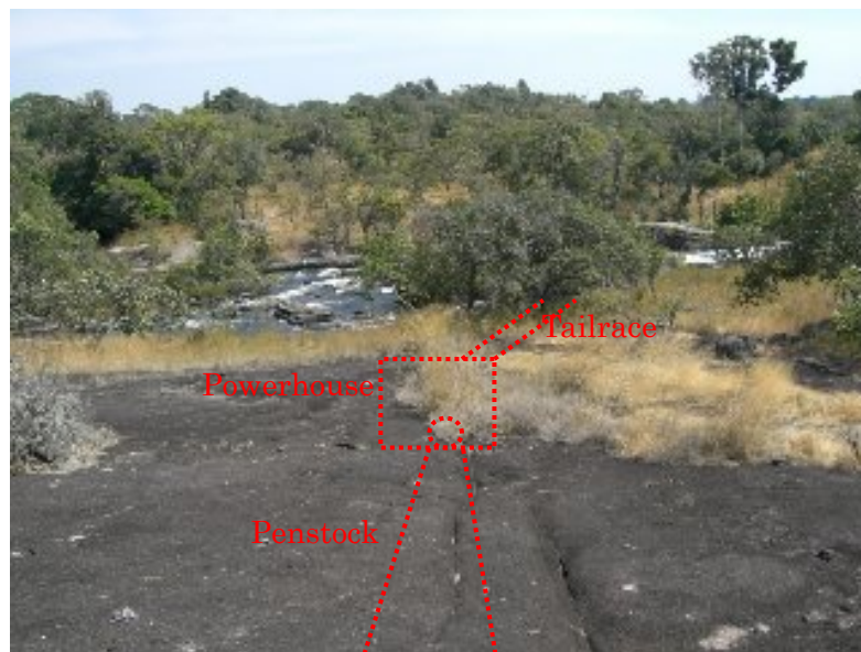
c) View from head tank to powerhouse
