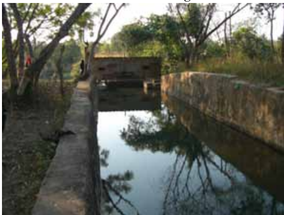
c) Water channel and powerhouse
