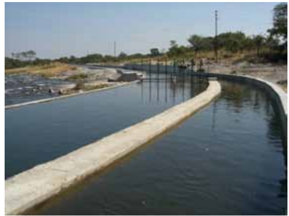
b) Silt basin and water channel
