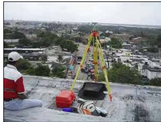
GPS observation at existing control point
