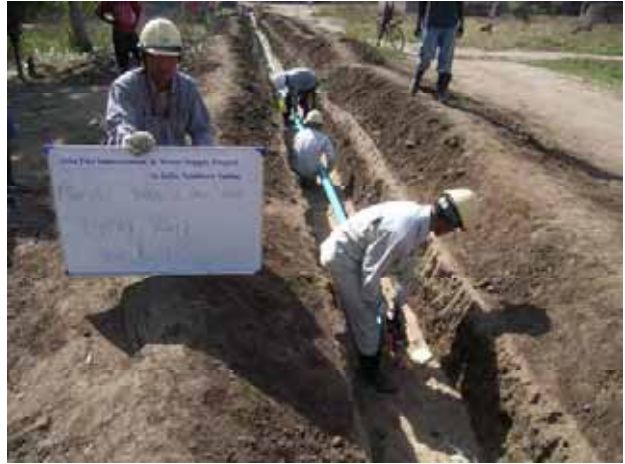
Distribution Pipe Line under Installation
