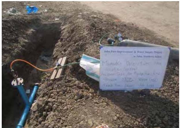
Pressure Test of Distribution Pipe Line
