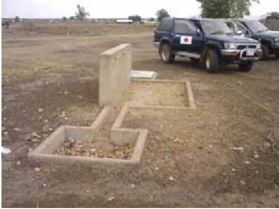
One of Hydrant
