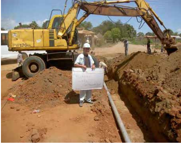
Transmission Pipe Line Under Installation
