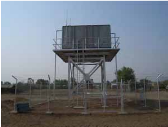
Completed Elevated Water Tank
