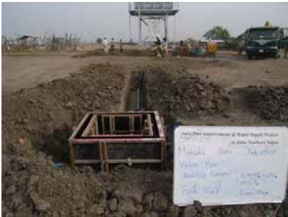
No1 Valve Box under Construction
