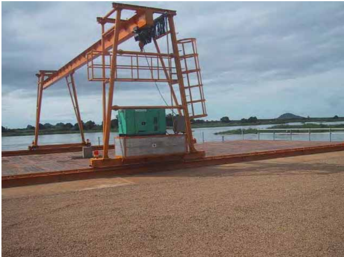
Port and Gantry Crane
