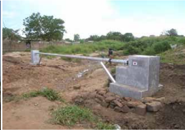
Water Pipe Bridge
