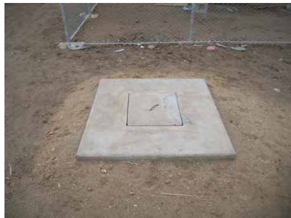
Drain Box for Elevated Water Tank
