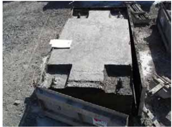
Removing Metal Form (May 10 th , 2007)
