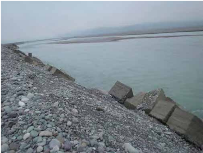
Temporary Installation of Concrete Block against Bank Erosion in BM 6.7km (December 2006)
