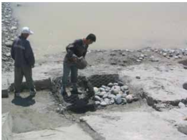
Rehabilitation of Existing Revetment Downstream of S1 (April 23 rd , 2007)
