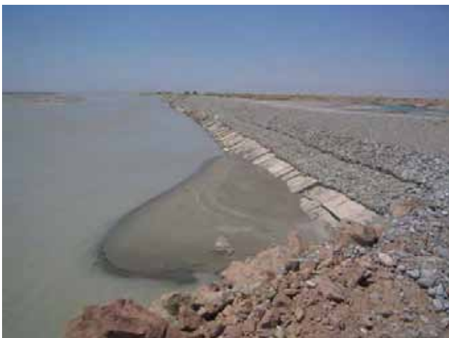
Combined Concrete Block and Gabion Type Revetment (July 2006)
