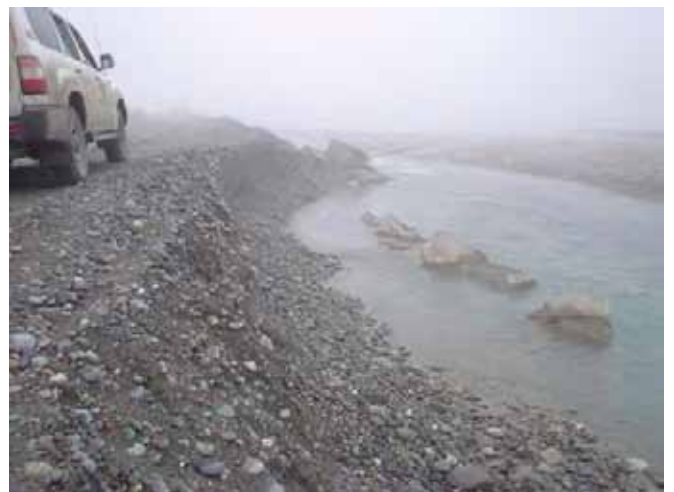
Temporary Installation of Concrete Block against Bank Erosion in BM 11.3km (December 2006)
