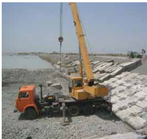
Slope Protective Work Downstream of S2 (May 3 rd , 2007)
