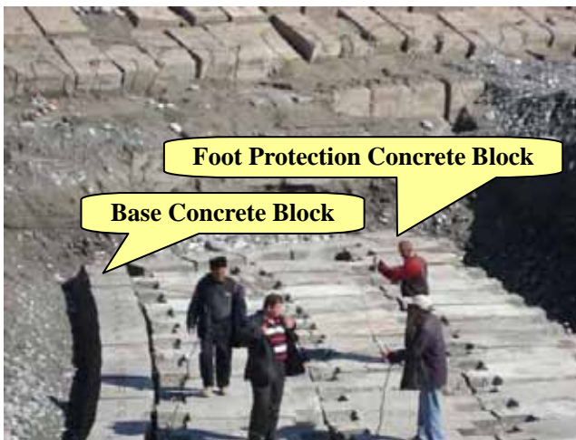
Base Concrete Block and Foot Protection Concrete Block in S1 (March 20 th , 2007)
