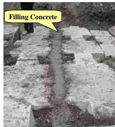
Filling of Spaces between Concrete Blocks in S2 (March 20 th , 2007)
