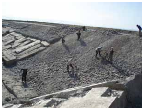
Trimming and Clearing a Slope Downstream of S1 (April 18 th , 2007)
