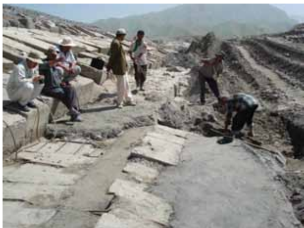
Filling of Spaces between Concrete Blocks on Revetment in Upstream of S1 (April 15 th , 2007)
