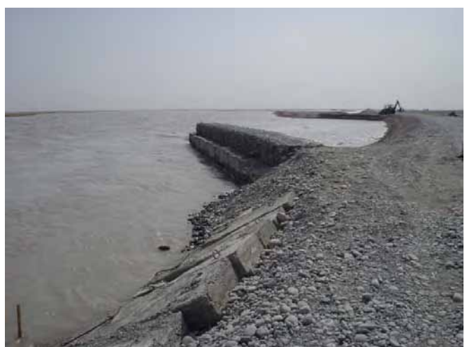
Concrete Block Spur Dike in Main Dike (May 2006)
