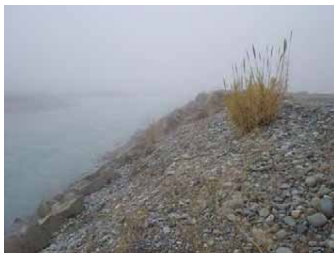
Revetment Washed Away in BM 3.0km (December 2006)
