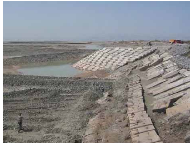
Slope Protective Work in S2 (April 10 th , 2007)
