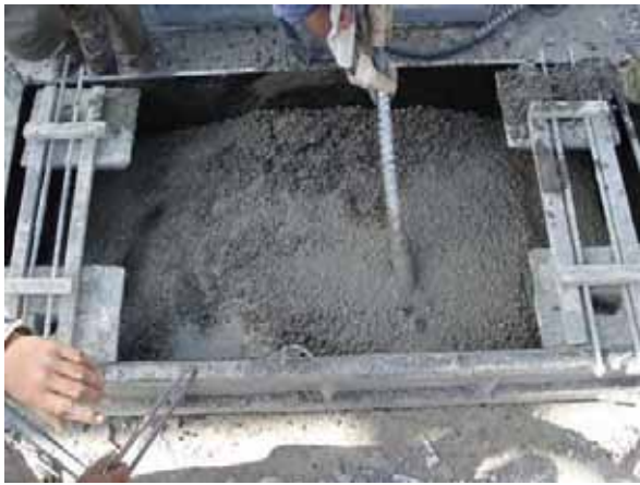
Compaction of Concrete (May 3 rd , 2007)
