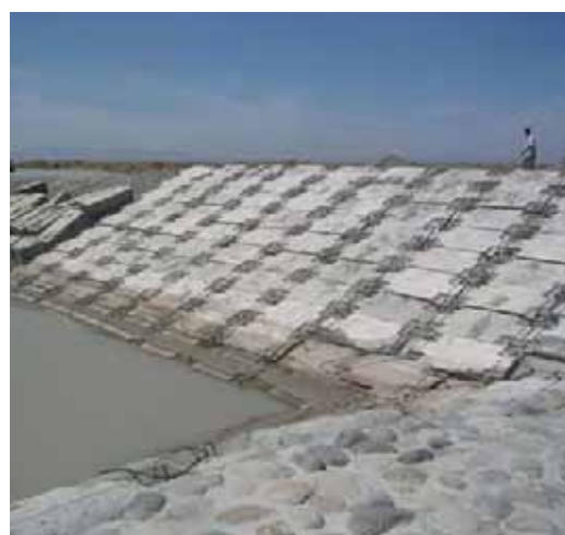
Slope Protective Work in Downstream of S2 (May 11 th , 2007)
