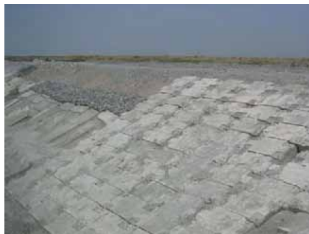
Slope Protective Work Downstream of S1 (April 28 th , 2007)
