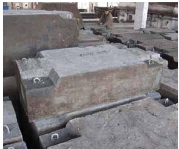
Completion of Concrete Block: 2.0m x 1.0m x 0.5m
