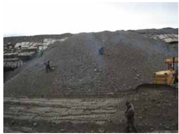
Trimming and Clearing a Slope in S2 (March 19 th , 2007)
