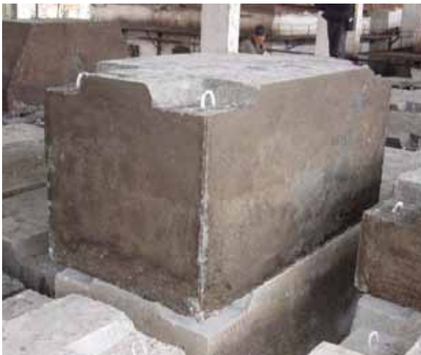
Completion of Concrete Block: 2.0m x 1.0m x 1.0m
