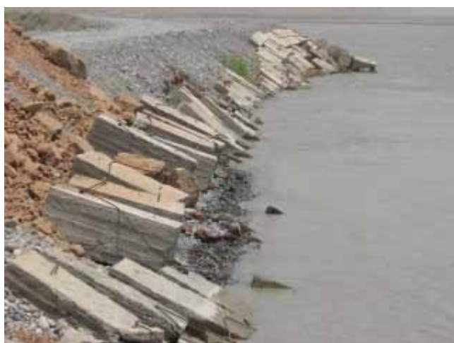
Temporary Installation of Concrete Block for Bank Erosion in BM 3.2km (July 2007)
