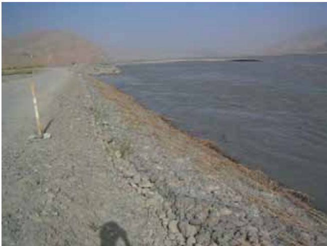
Gabion Type Revetment (September 2006)
