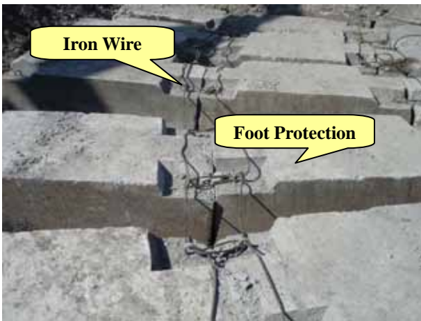
Connecting Concrete Blocks with Iron Wire in S2 (February 28 th , 2007)
