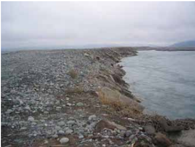
Temporary Installation of Concrete Block against Bank Erosion in BM 9.2km (December 2006)
