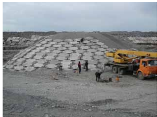
Slope Protective Work in S2 (March 24 th , 2007)
