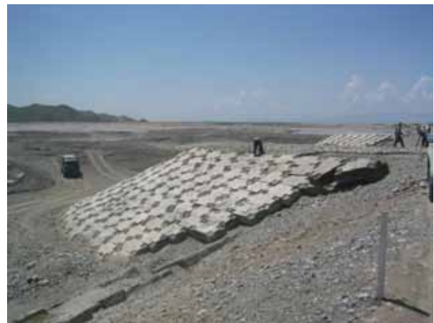
Slope Protective Work in S1 (April 23 rd , 2007)
