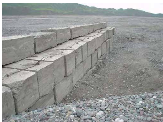
Concrete Block Spur Dike in Guide Dike (March 2006)
