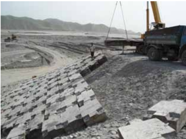
Slope Protective Work in S1 (April 16 th , 2007)
