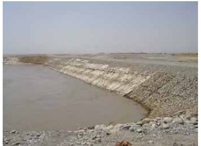
Concrete Block Type Revetment (August 2006)
