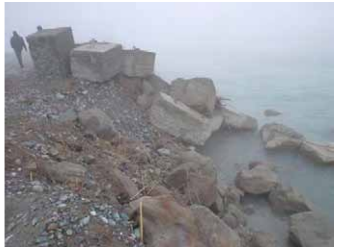
Temporary Installation of Concrete Block and Boulder against Bank Erosion in BM 10.3km (December 2006)
