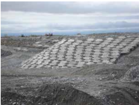
Slope Protective Work in S2 (March 30 th , 2007)
