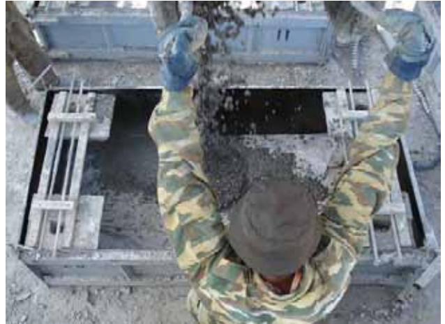
Pouring Concrete into Metal Form (May 3 rd , 2007)
