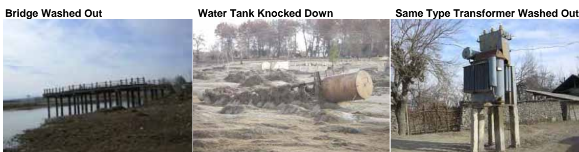
Fig. R 9.2.3 Some of Public Structures Damaged by 2005-Flood
