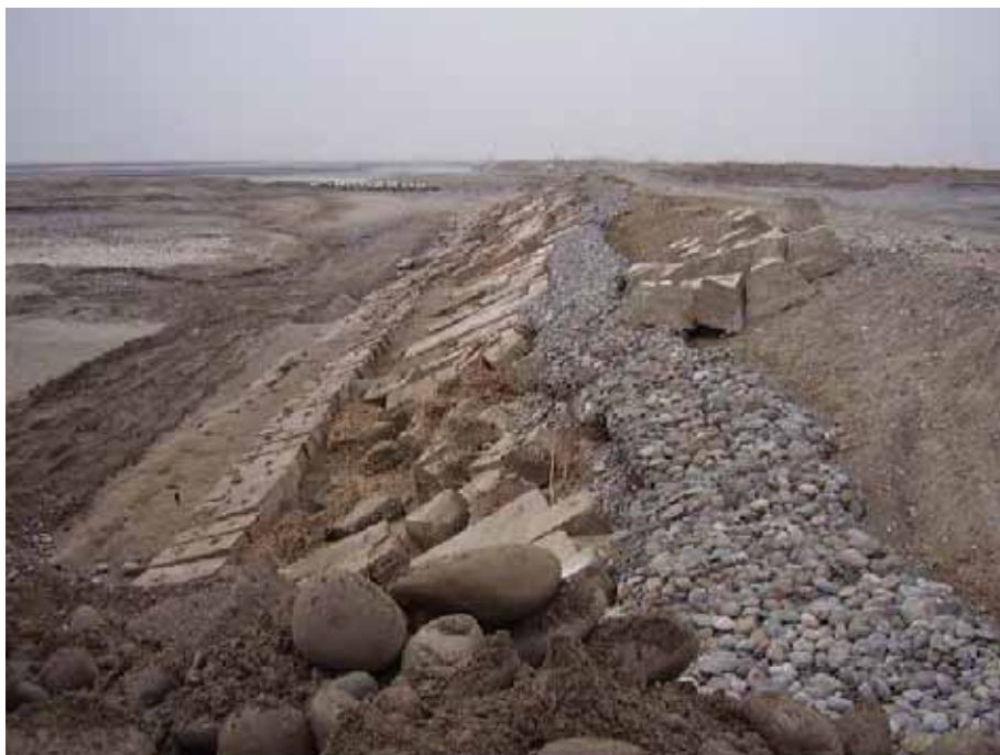
Fig. R.7.3.2 Dike Failure and Collapse of Blocks at Dike (River bank)
