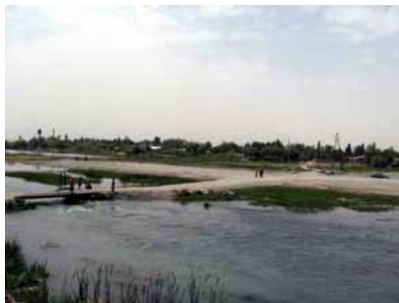
Fig. R 8.7.13 Temporary Bridge between Tagnob and Fayzobod
