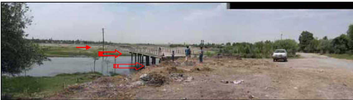
Main body of the Bridge (length 20.0 m, width 8.0 m) was not damaged by Flood
