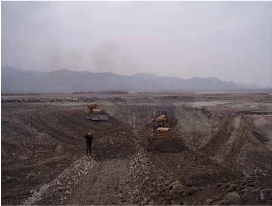
Fig. R.7.3.3 Machinery at Construction Site of Pilot Project
