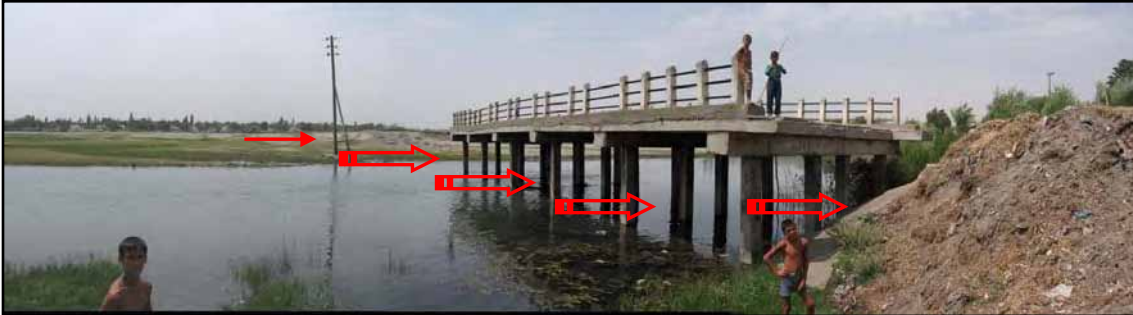
Main body of the Bridge (length 20.0 m, width 8.0 m) was not damaged by Flood
