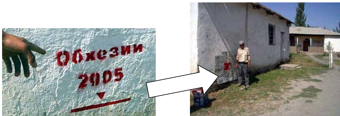
Fig. R 8.9.2 Indicator on the wall of the ex-post office in Dashti Gulo
