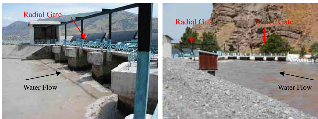
Fig. R 1.6.10 Photograph of Chubek Weir
