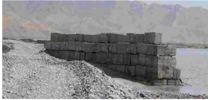
Fig. R 1.6.3 Photograph and Typical Design of Concrete Block Spur Dike
