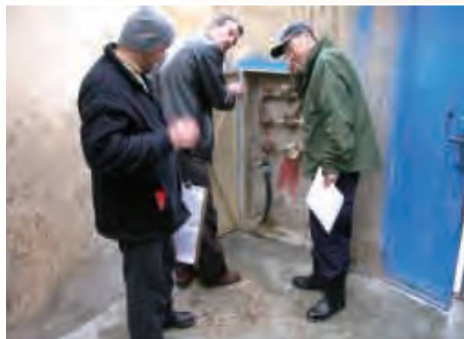
Checking a water meter using a listening stick
