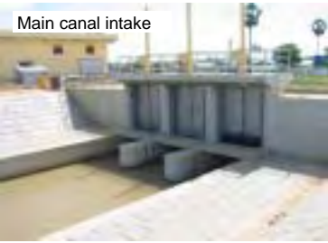
Main canal (complete)
