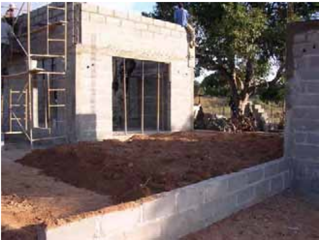
Masonry wall: Indoor Market Shed from patio side
