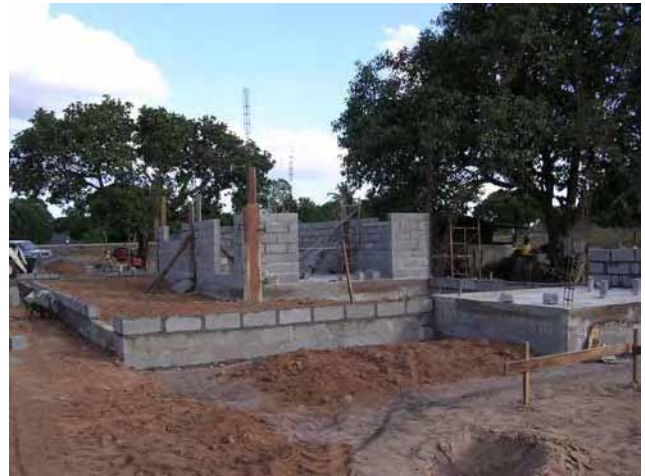
General view 2 (6/4) : public toilet side
