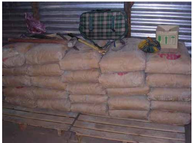
Delivered Cement materials
