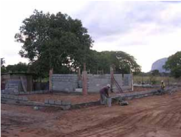
General view1 (6/4) : from terrace side
