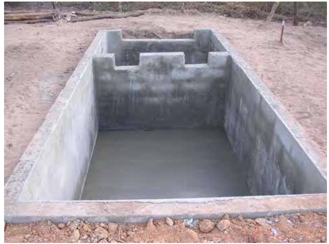
Septic Tank: side wall completed
