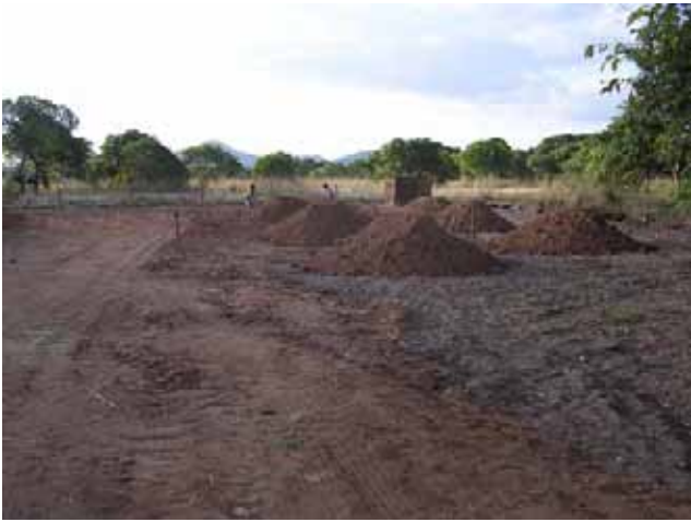
Parking Area: preparation borrow material for grading
