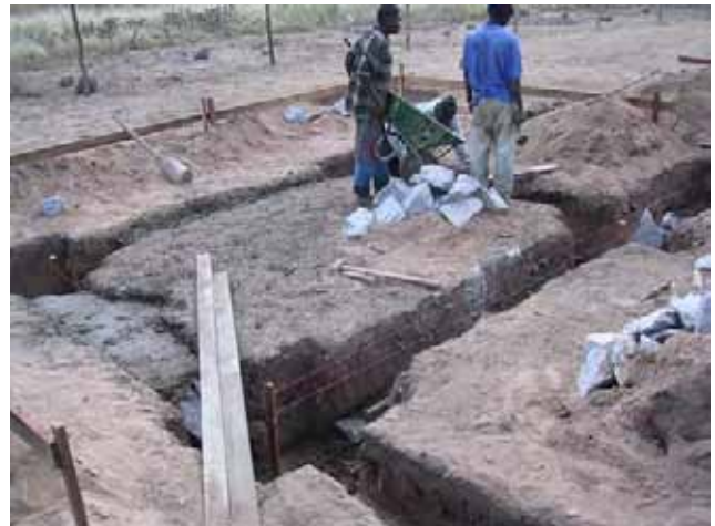
Foundation work: Public Toilet Shed excavation
