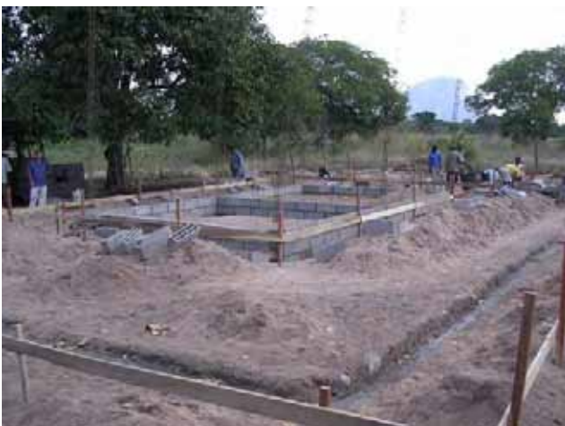
Foundation work: Public Toilet Shed completed
