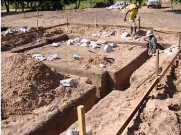
Foundation Work: Indoor Market Shed excavation
