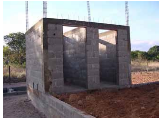
Masonry wall: Public Toilet from patio side
