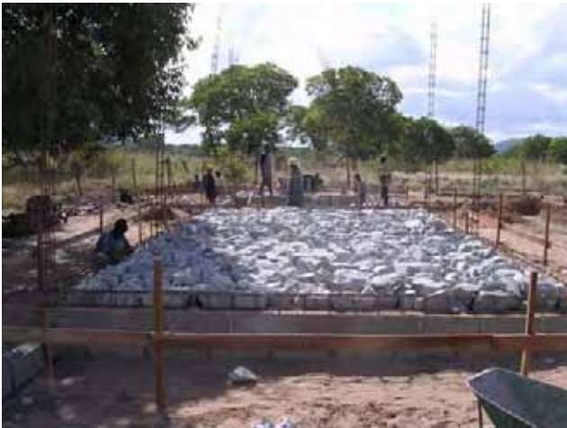
Floor concrete : Indoor Market Shed rubbles preparation
