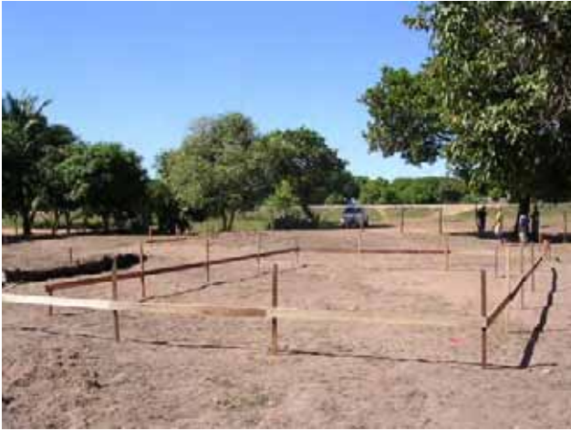
Setting out of the Building: Indoor Market Shed
