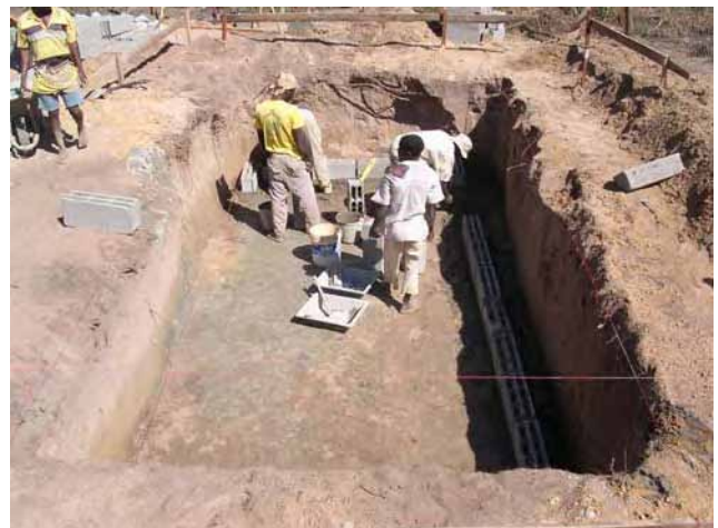
Septic Tank: excavation
