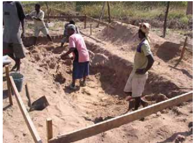
Septic Tank: excavation
