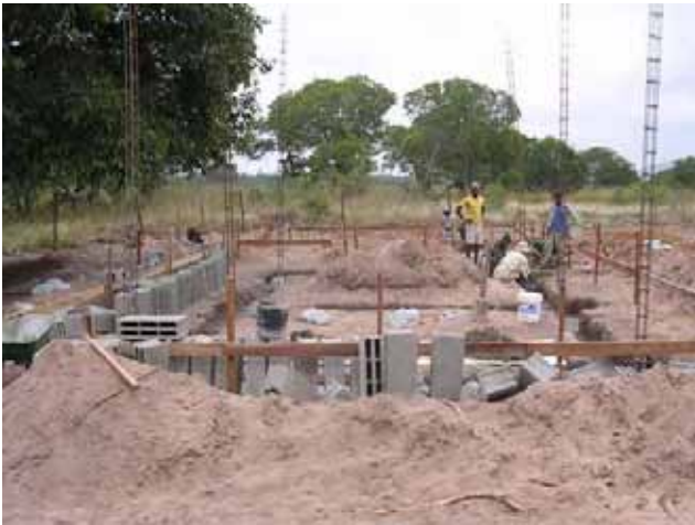
Foundation work: Indoor Market Shed view
