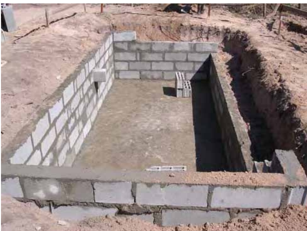
Septic Tank: wall masonry
