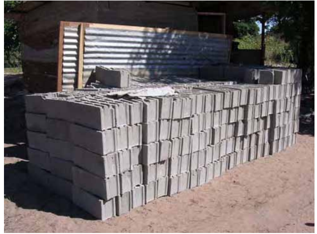
Delivered Concrete Block materials
