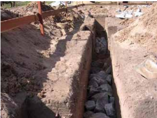
Foundation Work: Indoor Market Shed laid rubbles
