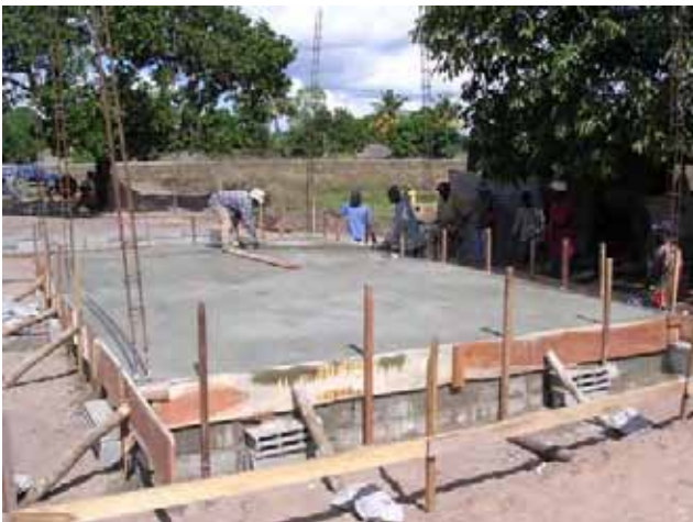
Floor concrete : Indoor Market Shed casting
