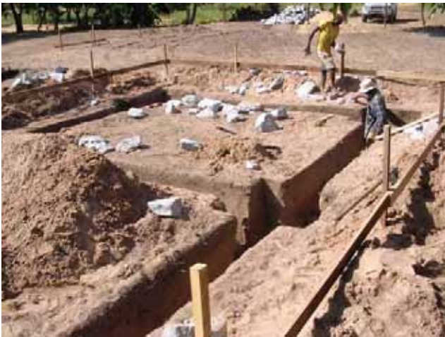
Foundation Work: Indoor Market Shed excavation
