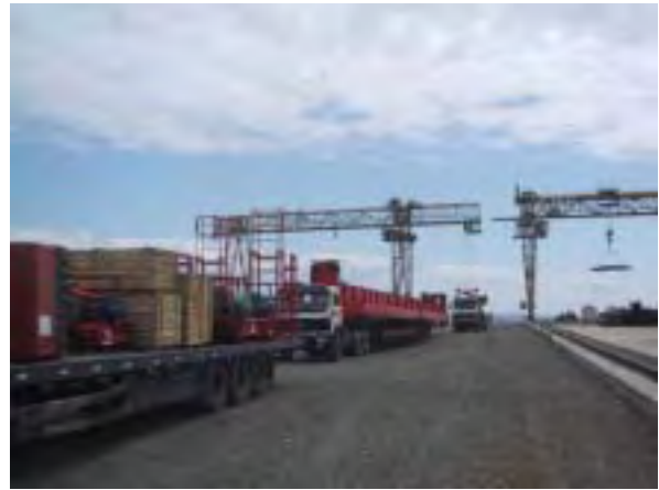
(Train Transfer Point No. 7)
