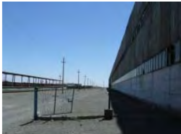
From the west: Northern side of loading and unloading facility No. 4
