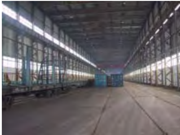
( Train Transfer Point No. 4)
