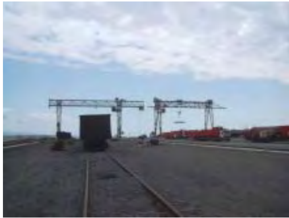
(Train Transfer Point No. 7)
