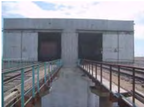
(Train Transfer Point No. 6, upper level)
