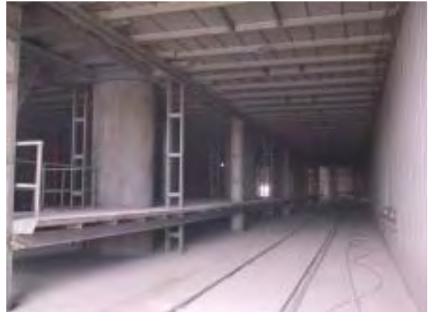
(Train Transfer Point No. 6, lower level)
