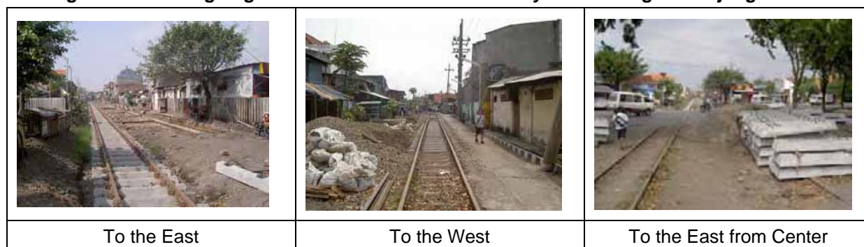
Figure 6.2.9 On-going Rehabilitation Works of Railway Track along Jl. Tanjung Perak
