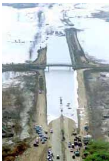
Toll road inundated by mud
