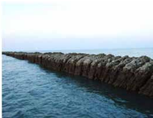
Figure 2.1.10 Present Condition of Existing Training Wall (12 June 2007)
