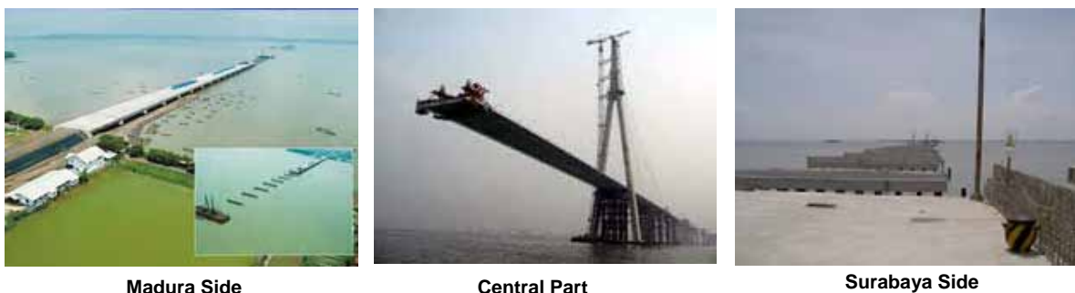
Figure 2.6 Progress of Sura-Madu Bridge Construction
