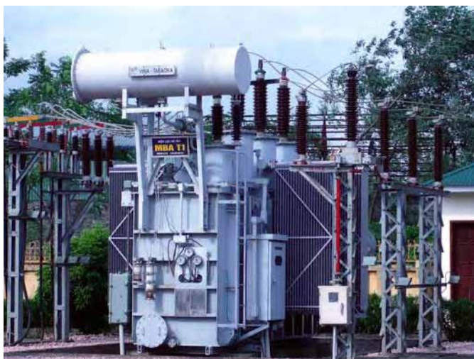
HHTP S/S Temporary Transformers ( 25MVA )
