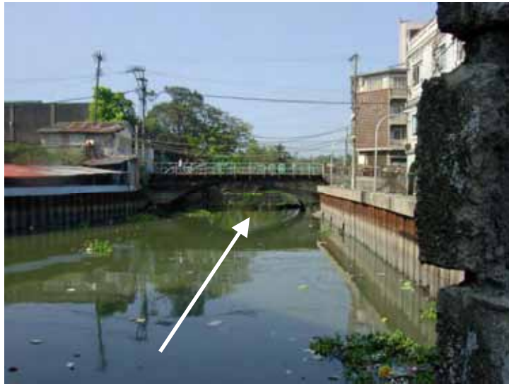
Downstream Canal of Quiapo Drainage Pumping Station as of March 3, 2007
