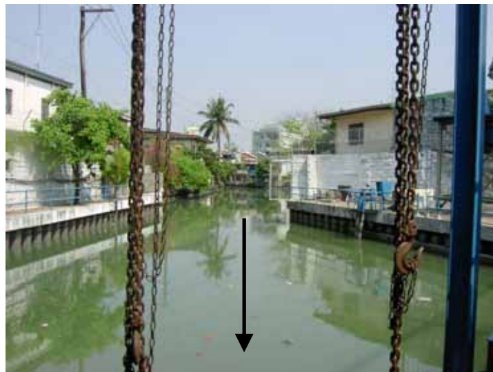
Inlet Canal to Aviles Sampaloc Drainage Pumping Station as of March 3, 2007
