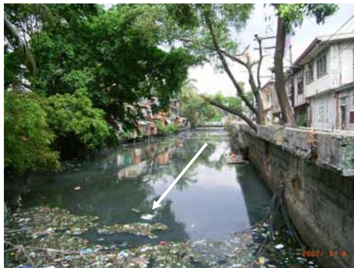
Secondary Canal to Estero de Quiapo as of March 8, 2007
