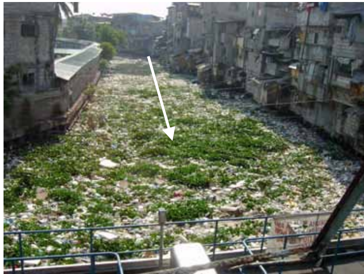
Inlet Canal to Quiapo Drainage Pumping Station (as of March 3, 2007)
