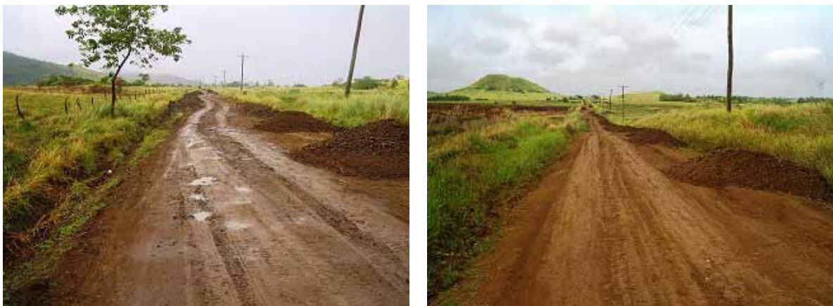
Figure 5-10 Existing Road Condition of Milagros – Balud Section
