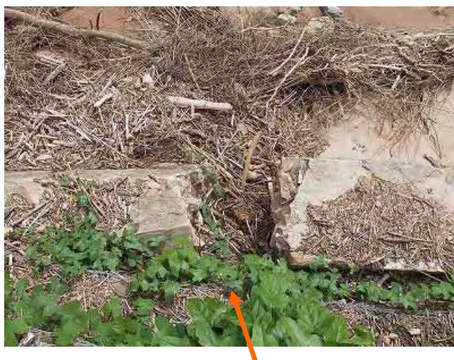
Photo 9.7.13 Opening of retaining wall by lateral compression
