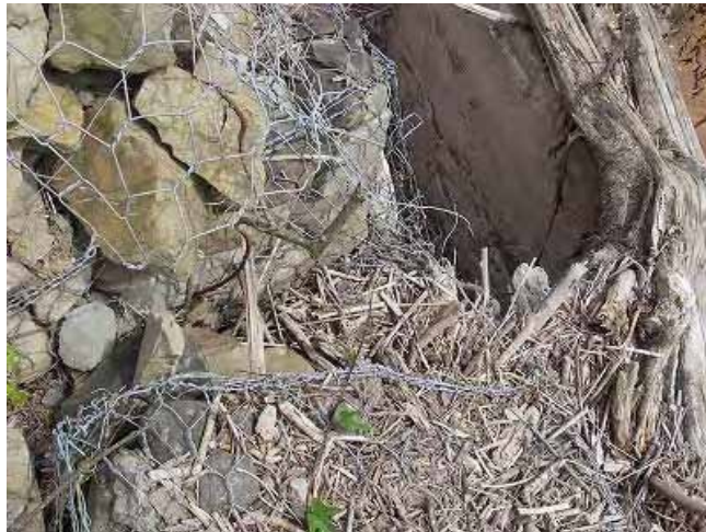
Photo 9.7.12 Opening of gabion by lateral compression
