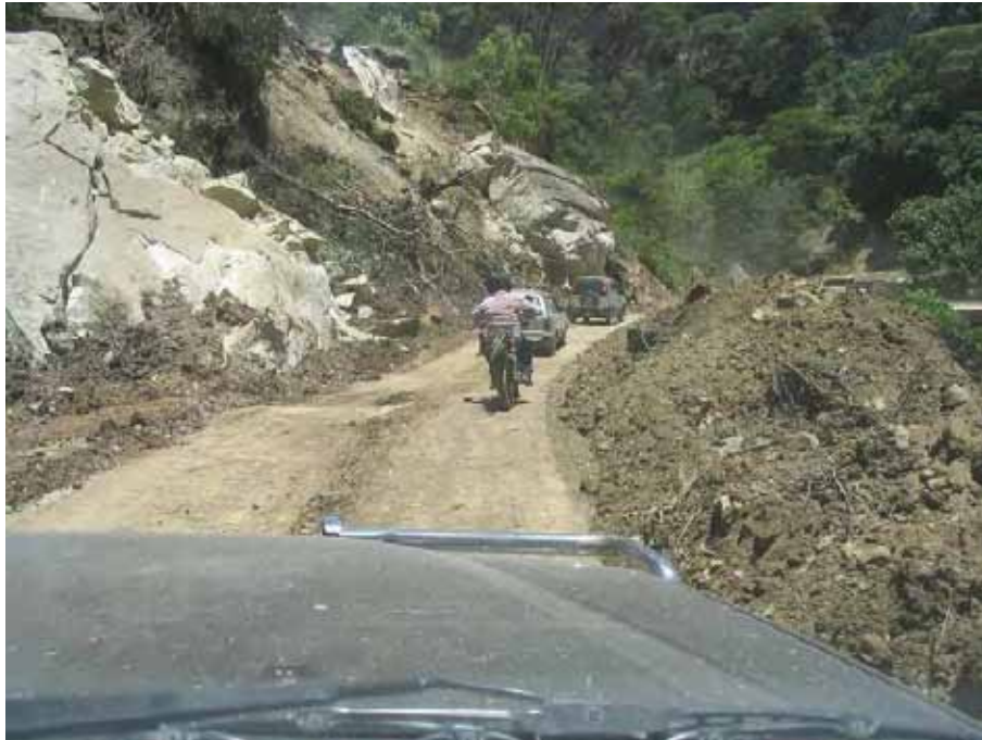
Photo 9.13.5 Site of rockfall
