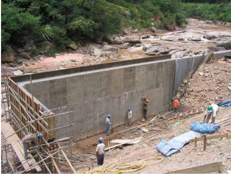
Photo 9.13.7 River revetment work (inverted T-type retaining wall under construction)
