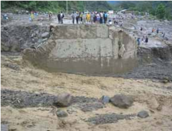
Immediately after the Tiyumayu Bridge disaster
