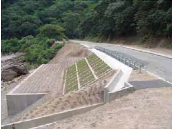
Pilot Works after Completion (March 2007)
