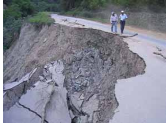
Collapse of Road Caused by Rain Water Bermejo, SCZ on Route 7 (February 2007)
