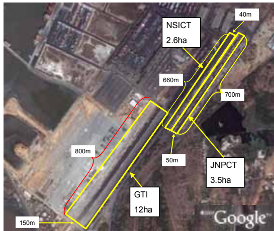
Figure 8-2 Rail yard of JNP at present
