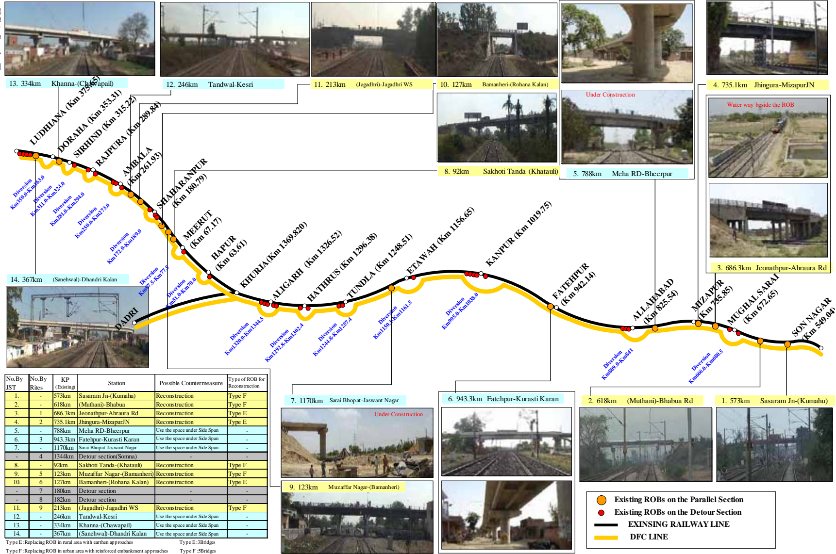
Figure 7-22 Existing ROBs on the parallel section on the Eastern DFC
