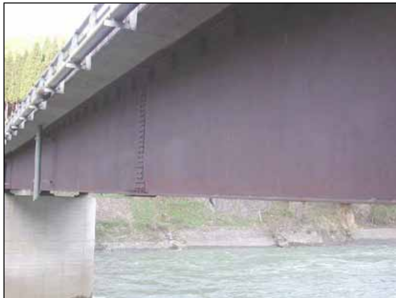
Figure 8-13 Bridge using Atmospheric corrosion-resistant steel
