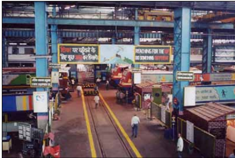
Photo 4-1 Vadodara Electric Loco Shed
