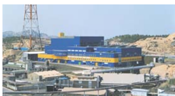
Intermediate Treatment Plant
