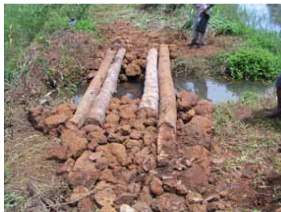
Wooden Bridge Constructed
