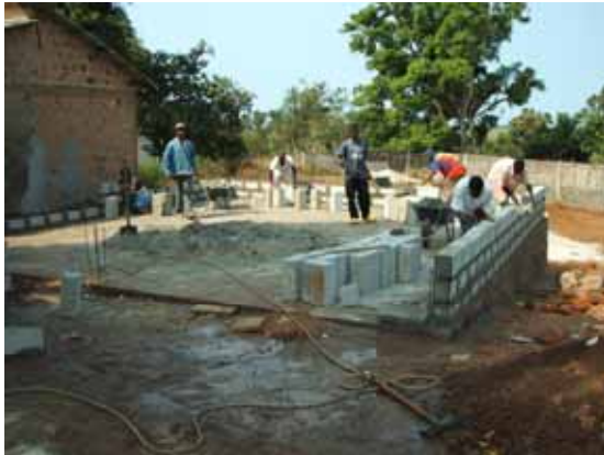
Shed under Construction
