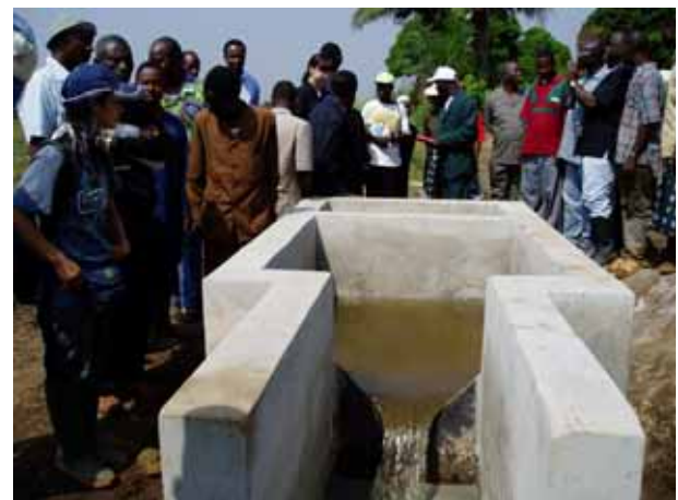
Basin with Triangular Weir (Small-scale Irrigation)
