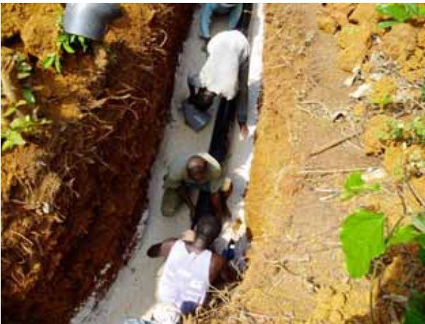
Pipe Installation (Small-scale Irrigation)
