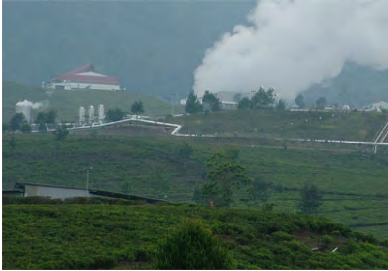
Fig. 7.4.4-2 Wayang Windu Geothermal Power Plant Located in Tea Plantation
