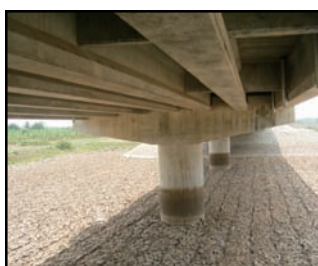
橋梁下面と護床工
