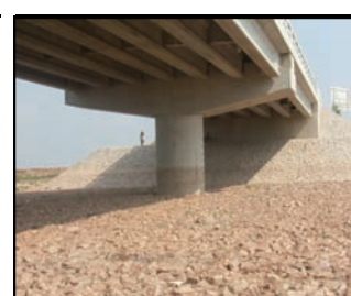
橋梁下面と護床工
