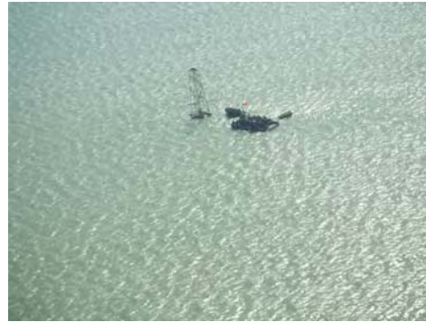
Shut off works of abandoned underwater well
