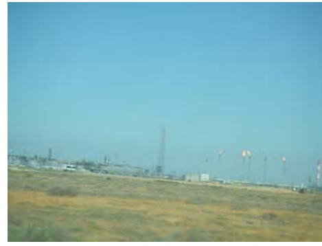
Flare stack of oil &amp; gas refinery
