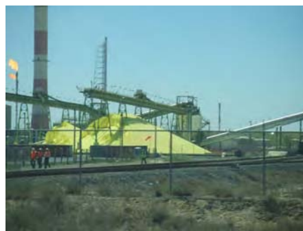
Shipping facility of granular sulphur
