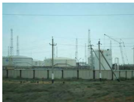
Open (Vent) type tank
