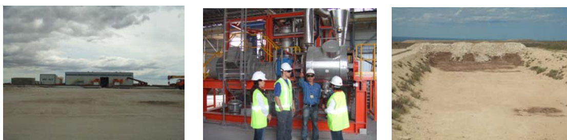
(new treatment building) (new thermal treatment facility) (disposal site of treated cuttings)
