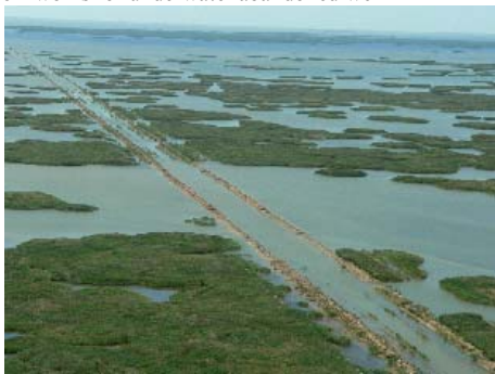
Construction of oil pipeline from Kashagan oil field
