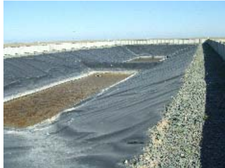
Construction of an industrial waste disposal facility
