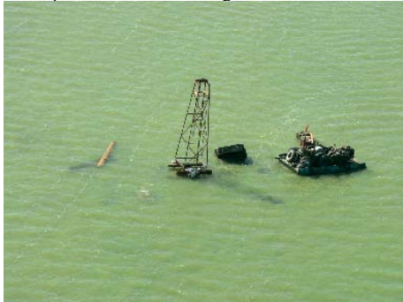
Shut-off works for underwater abandoned well
