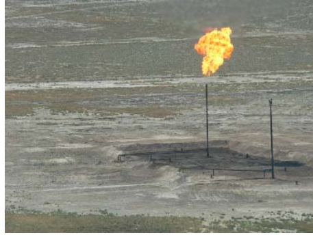
Condition of flare
