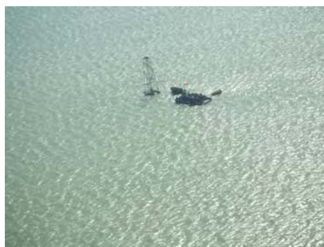
Shut off works of abandoned underwater well
