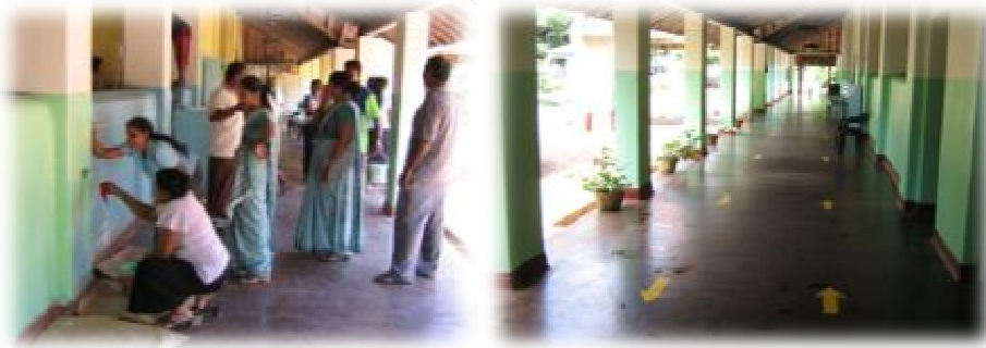
FIGURE 5- 3: CLEANING AND PAINTING THE CORRIDOORS
