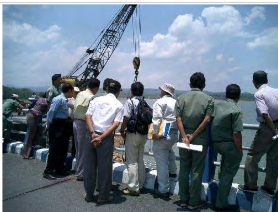
Counterpart Meeting on October 3, 2005 (site inspection for verification test of hydro-suction system)
