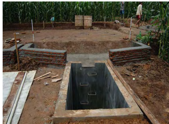
Construction of water tank and farm field at Slogohimo site
