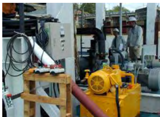
Equipment on barge on October 12, 2005
