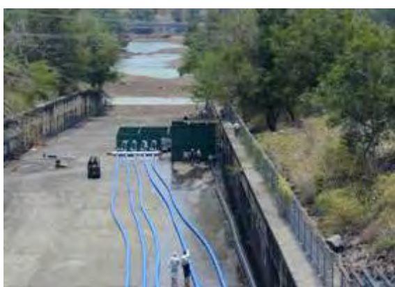
Examination of the appearance of Return-to-Reservoir Pipe on October 11, 2005
