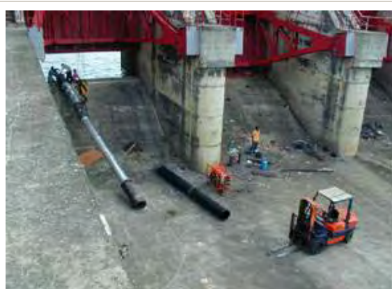
Placing steel pipe at spillway crest on October 4, 2005
