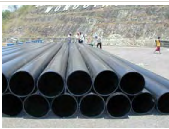
High-density polyethylene pipe (Φ 400) for dredging pipe on September 26, 2005
