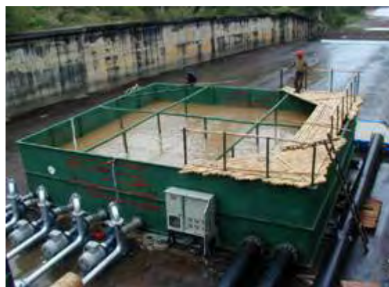
View of storage tank on October 24, 2005
