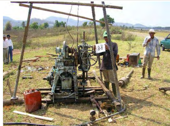
Drilling at the location of proposed overflow structure
