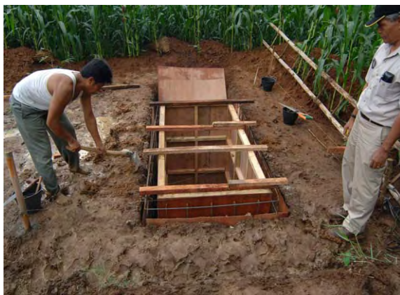
Construction of water tank (casting concrete) at Slogohimo site
