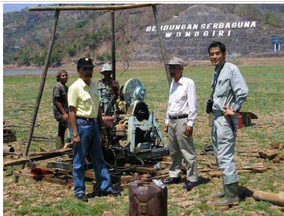
Drilling at the location of proposed closure dike
