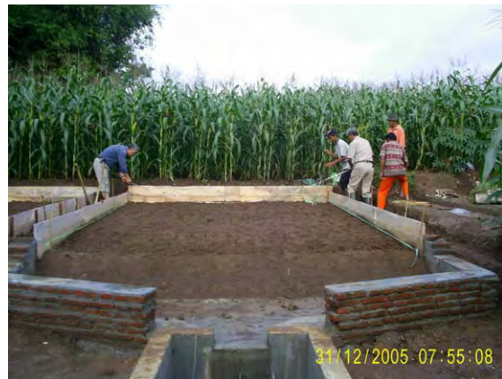
Construction of water tank at Sologohimo site
