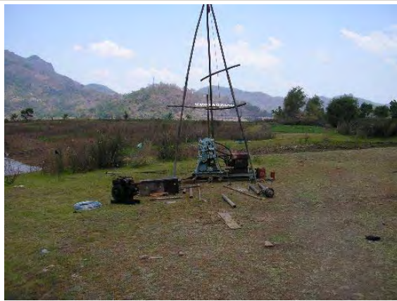
Drilling machine for geological investigation on October 2006
