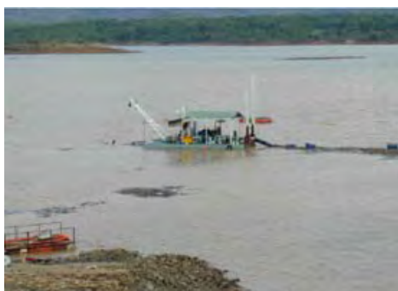
Verification test of hydro-suction system at intake on October 19, 2005
