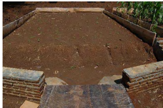
Terrace with bare land condition on February 19, 2006
