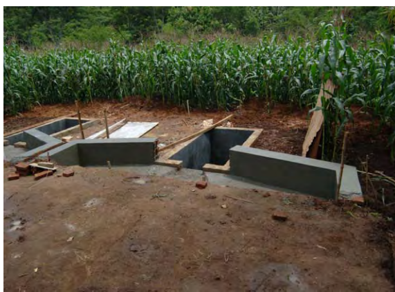
Construction of water tank at Sologohimo site
